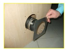
5.) Push the second flange plate on the tube. The eight lugs must be under the hose clamp.
